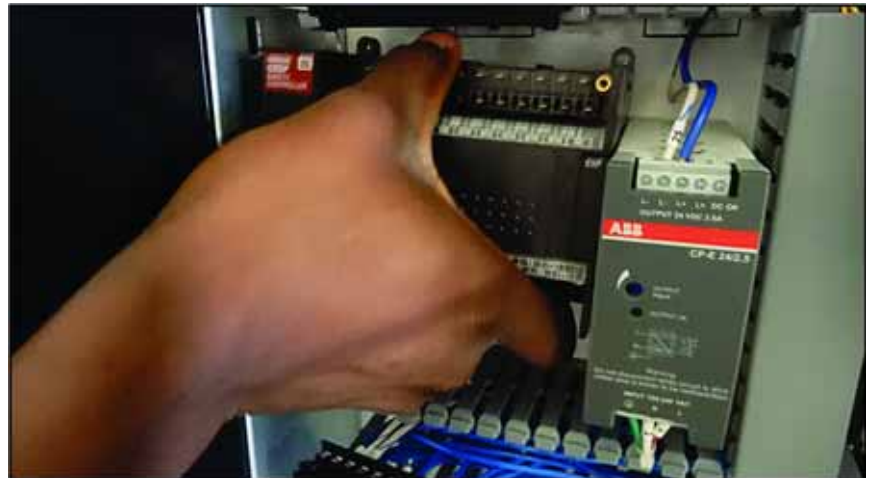
Figure 8: Removing the Safety Controller
