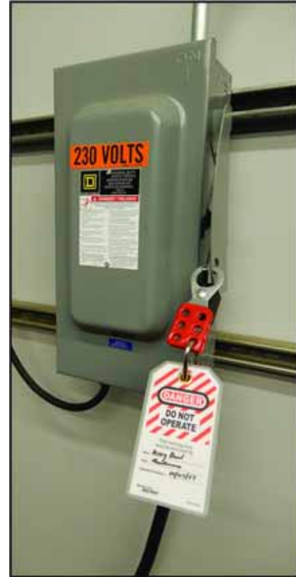
Figure 3: Lockout/Tagout on the Electrical Service Entry Panel
