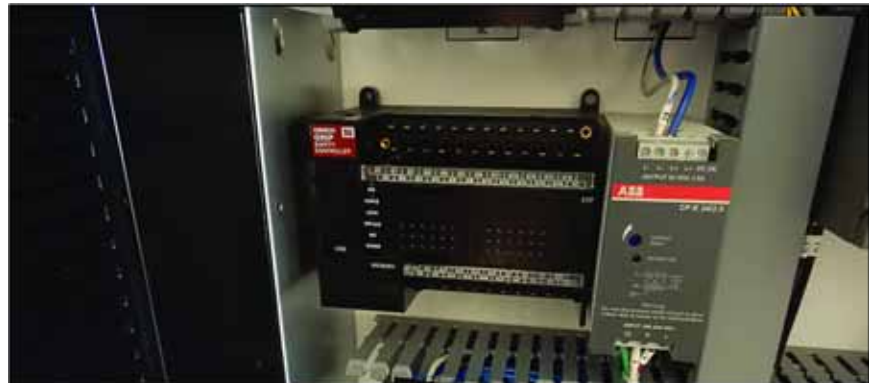
Figure 6: Input and Output Terminal Blocks Removed
